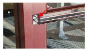
East automatic doors have pin-type hinges which can loosen, making the door fall off (potential safety hazard) if the adjusting screw is not periodically inspected and kept tight.
