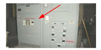
SWBD 1 is a secondary main panel, 1000 amps, 480/277 volts, 3Ø, fed from swbd2 on an 800 amp circuit breaker. It has its own disconnect handle on the panel itself.
