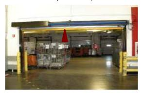
Interior Lighting System: Most interior lighting is low-energy, high efficiency 277V fluorescent, consisting of high-mounted walkway illumination, with lower-mounted task lighting fixtures. These lights are controlled by the computer (Polaris program) in the "maintenance' office. The program instruction book was located by the computer on the day of the inspection. A few lamps were not working on the day of the inspection. A few lights are incandescent. Lighting appears to be adequate.
