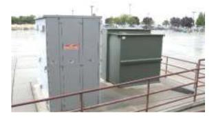
Switchboard (swbd) 2 is the main panel for the building. SWBD 2 has the main service disconnect (push button type), is rated at 2400 amps, 480 volts, and has a phase detector.
