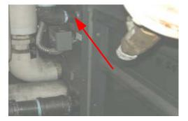
AH 4 (19,000 CFM) serves the east and middle docks, plus the customer area and personnel offices on the east end of the building. Supply fan drive motor is 3phase, 460V, 15hp, with a Cutler-Hammer HV 9000 variable frequency drive; has a 3-way valve on the chilled water line.
