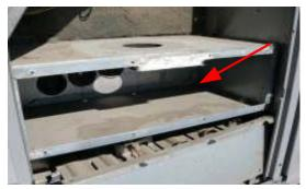
The medium-sized RTUs have wires that are located such that they can be damaged when sliding the filter carrier during filter changes. Maintenance personnel will need to be cautious.
