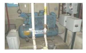
Ingerson-Rand rotary air compressor Single motor; 30hp, 3Ø, 460V Automatic condensate relief valve on tank and lines has small oil leaks Has air dryer Safety Issue: No record of a recent "unfired pressure vessel" pressure test.
