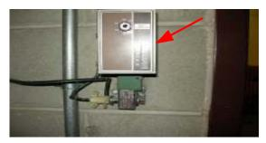
The boiler emergency shutoff buttons are located outside the north mechanical room door, and on the wall inside the mechanical room by the south exit door
