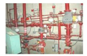
The fire sprinkling system consists of one dry pipe system and three wet pipe systems, all "supervised" (monitored) by the Delta 90 fire alarm panel. The sprinkling systems were last inspected by a professional company in March 2006. Records of the previous occupant indicate that the system has been inspected yearly. No problems were visible on the wet pipe systems.
