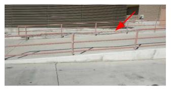
The faded paint on the step-down ledge in the truck parking lot requires repainting for safety visibility.
