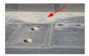
The roof infrared (thermal imaging) scan performed in March 2011 indicated a few minor problems; the results are on file in the maintenance office. There appears to be a little wet insulation under the membrane in one spot.
