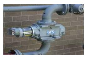
Some gas piping has deteriorated paint (left photo). Some gas piping standoff blocks on the roof are deteriorated or missing (right photo).
