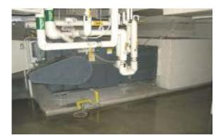
AH 3 (11,400 CFM) serves the east half of the east workroom floor. supply fan motor is 3phase, 460V, 7.5hp, with an ABB variable frequency drive (2011). AH 3 shows evidence (plumbing pipes) of the hot water coil having been replaced (2011)
