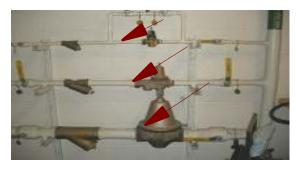
A backflow preventer to prevent a cross-connection between the potable water distribution system and the non-potable water is located in mechanical room; it was tested May 2011. Test the backflow preventer yearly.
