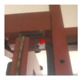
A representative number of windows was inspected: most windows are dirty most have venetian blinds on the inside fading paint on window frames some water stains on frames no signs of leakage
