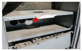
The medium-sized RTUs have wires that are located such that they can be damaged when sliding the filter carrier during filter changes..
