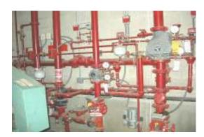
The fire sprinkling system consists of one dry pipe system and three wet pipe systems, all "supervised" (monitored) by the Delta 90 fire alarm panel. The sprinkling systems were last inspected by a professional company in March 2006. Records of the previous occupant indicate that the system has been inspected yearly. No problems were visible on the wet pipe systems.
