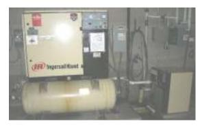
Air lines (steel and copper) with quick connectors and shutoff valves are distributed throughout the building and to the outside on the south side. No leaks were noticed. An ultrasound test can find small leaks that may otherwise go unnoticed.
