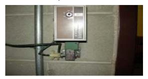
The boiler emergency shutoff buttons are located outside the north mechanical room door, and on the wall inside the mechanical room by the south exit door
