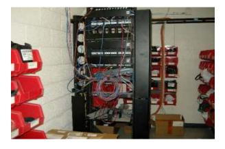
The public address (PA) system is located in the "supervisors' office" on the north side of the building. Speakers are mounted throughout the building and were working on the day of the inspection.
