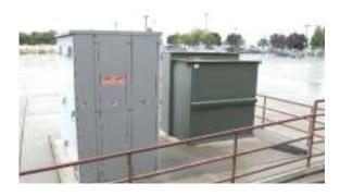
Switchboard (swbd) 2 is the main panel for the building. SWBD 2 has the main service disconnect (push button type), is rated at 2400 amps, 480 volts, and has a phase detector.
