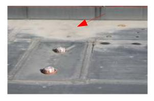
Roof Infrared Scan – performed March 2011; few problems; results are on file in the maintenance office. There appears to be a little wet insulation in one spot
