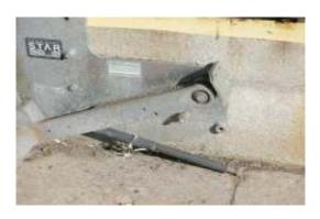
The swinging arm truck loading lights are operational; some lamp guards are missing. There were no exposed exposed electrical hazards, except for loose lens and no lamp guard on the trailer light by the compactor.
